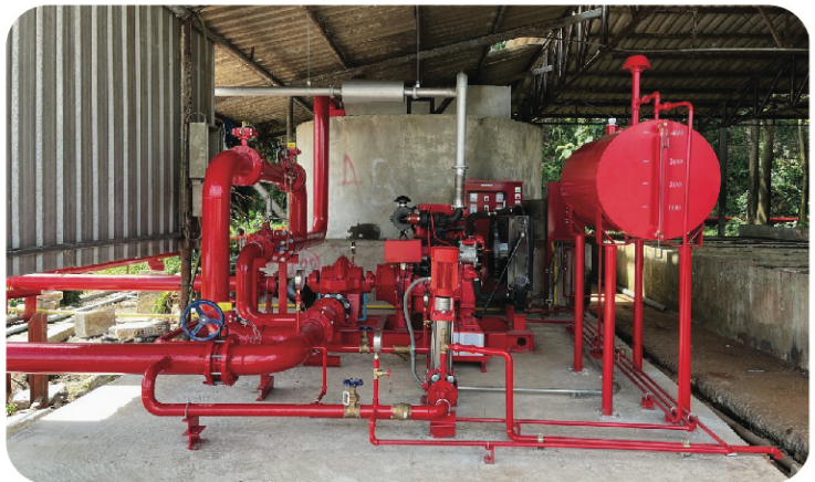
Replacing fire pump and fire pipe as per NFPA Standard
